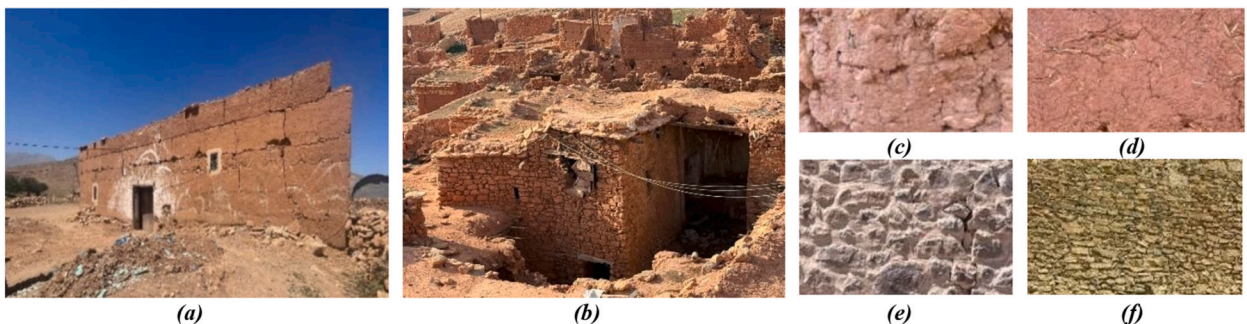
Fig. 17. URM typologies (a) RE; and (b) SM. Construction details: (c) RE with gravels and small pebbles; (d) RE with straw; (e) rounded SM; and (f) flat SM.
