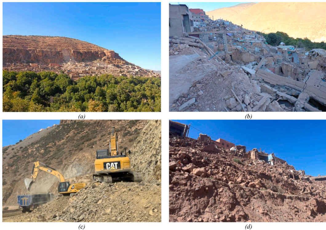
Fig. 2. Earthquake impacts in the High Atlas region: (a) overview of Imi N'Tala Al Haouz Province (High Atlas Mountains), showing a typical mountain settlement with dense construction along steep slopes; (b) extensive collapse of residential buildings in Imi N'Tala, constructed with non-engineered techniques in remote communities; (c) earthquake-triggered rockfalls and landslides along the Tizi N'Test corridor, obstructing mountain roads and requiring clearance operations; and (d) collapse of hillside dwellings in Talat N'Yaaqoub, illustrating the interaction between steep terrain and structural vulnerability.
