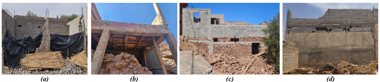
Fig. 25. Temporary shelter: (a) Confined Masonry (CM) with Concrete Masonry Units (CMU) panels without first-floor slab; (b) CM with stone masonry (SM) panels with traditional floor. Intermediate Housing: (c) CM with SM panels with a reinforced concrete (RC) sill band enclosing short CMU, (d) CM with CMU panels without the sill band.
