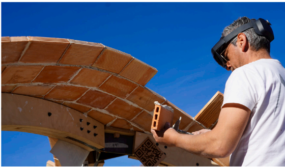
Fig. 3. Augmented thin-tile vault construction using digital guidework.
