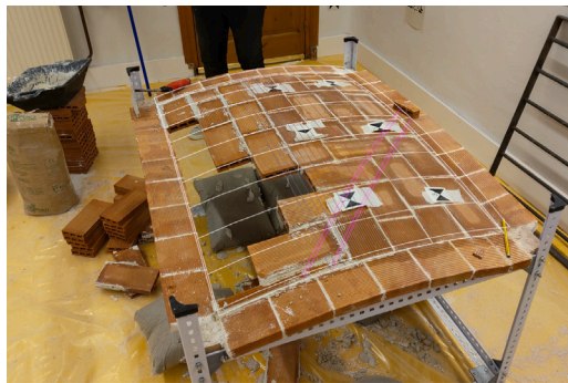
(a) Small vault built in lab environment
