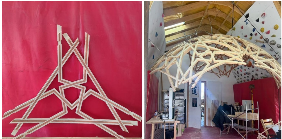
Fig. 18 The process of assembling the spherical triangles in the workshop. Left, a typical spherical triangle. Right: assembling part of the pavilion
