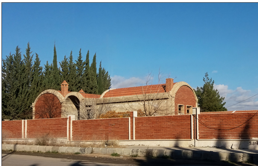
Figure 18: Al-Sharqyat today. Reformed house with extensions and covered vault with terracotta tiles. Photo by Wesam Al Asali.
