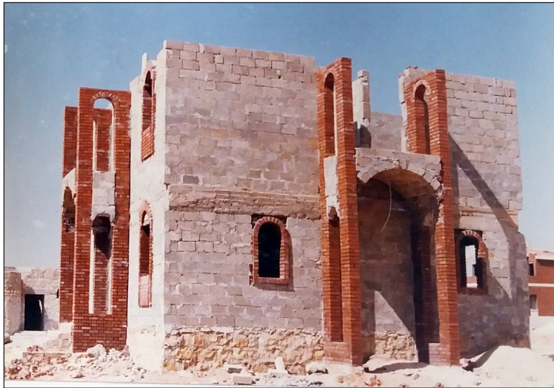
Figure 12: Construction of first experimental houses in Al-Sharqyat using local materials. Source: Mousally (1988: 98).
