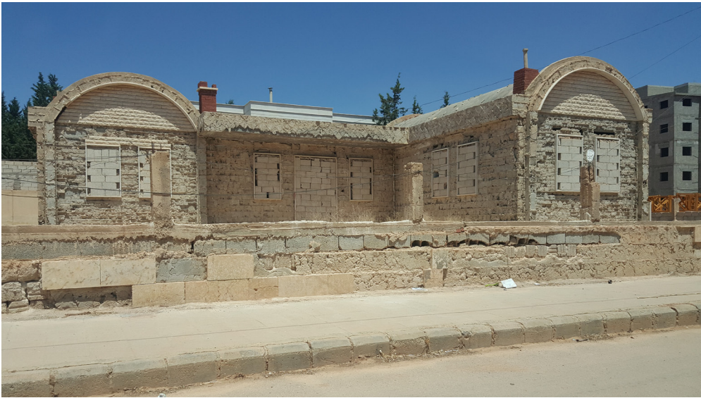
Figure 17: Al-Sharqyat today. Abandoned house, as built by Milihouse in 1990s, without its mortar finishing and showing the original material of cement block. Photo by Wesam Al Asali, 2019.
