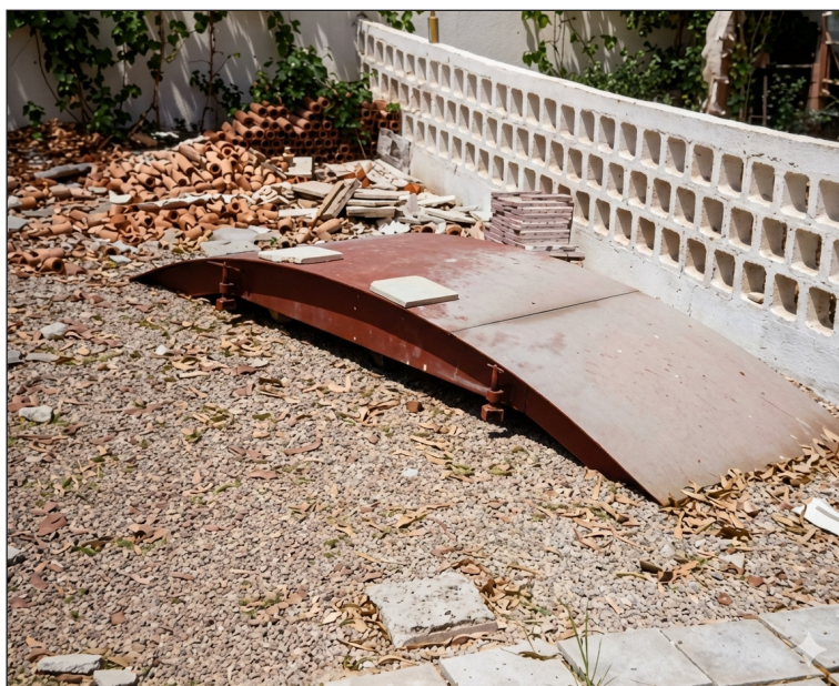
Figure 9: Solutions for vaulted structures at Damascus Expo, 1981: Sliding formwork and terracotta tubes prepared for the shallow vaults floor-systems for rural housing, made by architects from the Faculty of Architecture in Damascus University. Source: Archive of Maen Abaza, 1984.
