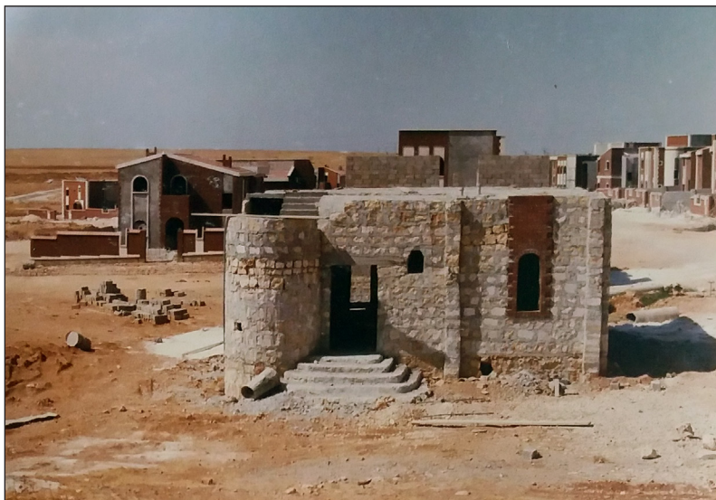
Figure 13: Construction of first experimental houses in Al-Sharqyat using local materials, and vaults for the second floor. Source: Mousally (1988: 99).
