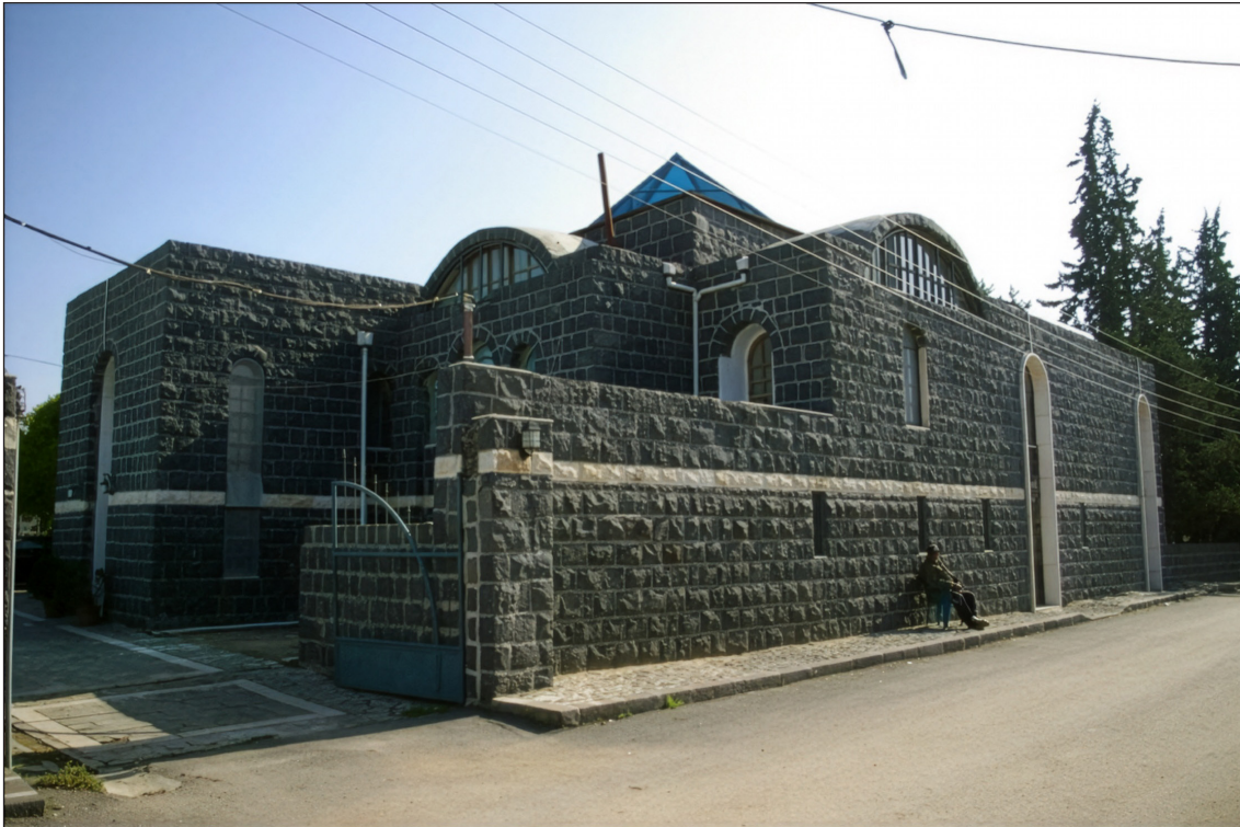
Figure 4: The vaulted system of basalt stone, developed by the Mouhanna brothers (Raef, Ziad, and Rafee), is here applied to a house they designed in As-Suwayda, Syria, in the late 1980s. Source: Archive of Ziad Mouhanna, 1988.
