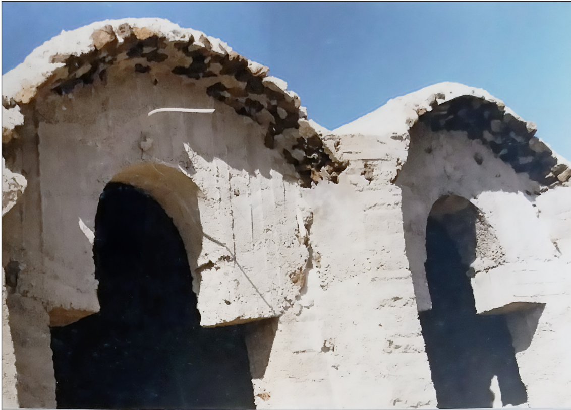
Figure 2: This rural house in Syria, built between 1987 and 1988 by Khaled Al Fahham, is of stone and cement vaults. Source: Mousally (1988: 84).
